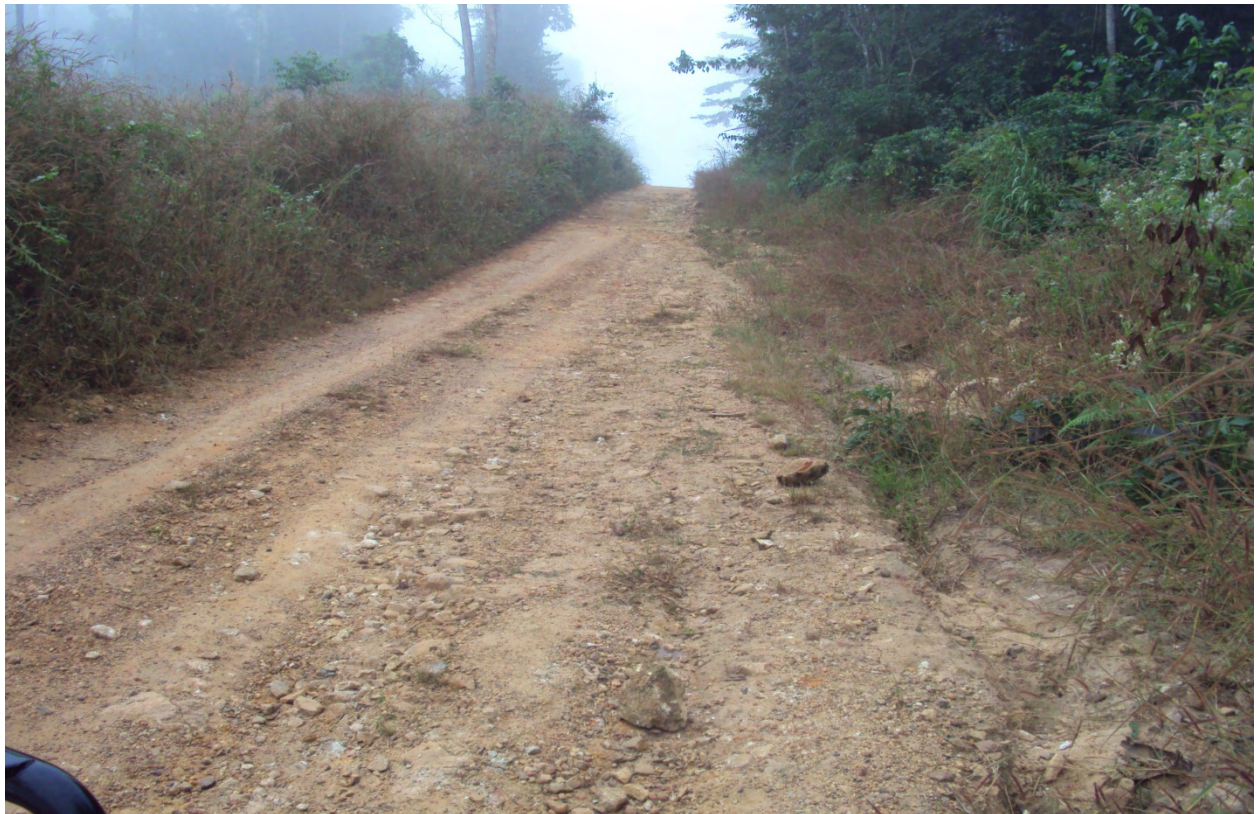
A hill going from Sengema to Sandaru shows erosion caused by the down hill rush of water.
