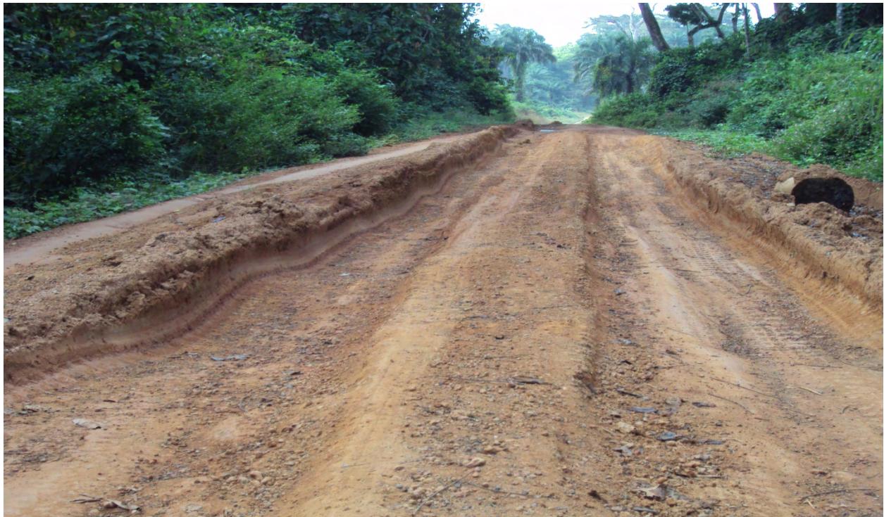
Looks bad, but a good surface -- ditching, re-grading and a roller will fix this.
