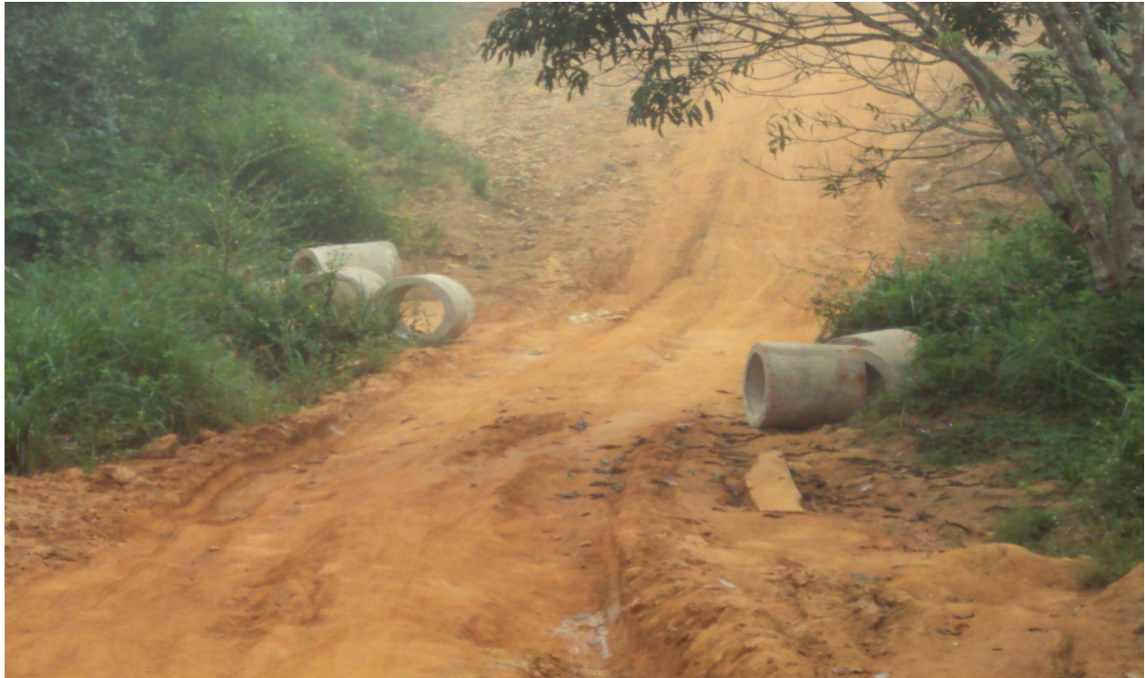
Culverts prepositioned by SLRA. Note the forest canopy over the roadway -- this keeps the road from drying, thus trees will be cut back in such areas.
