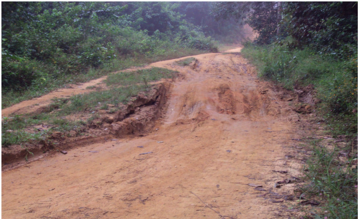
Fill, grading, new ditching and roller work is needed here.
