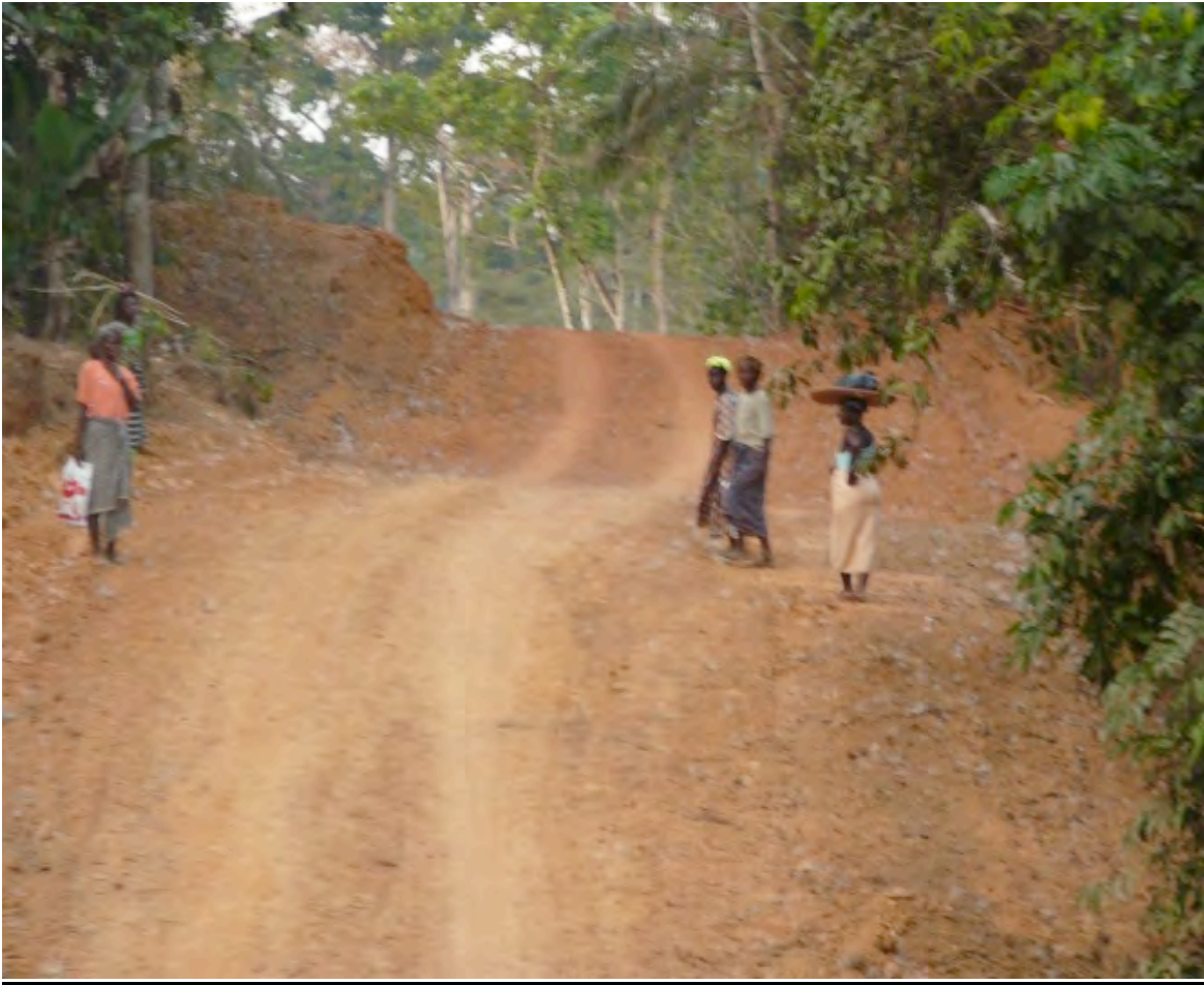
Cleared to Sandaru
