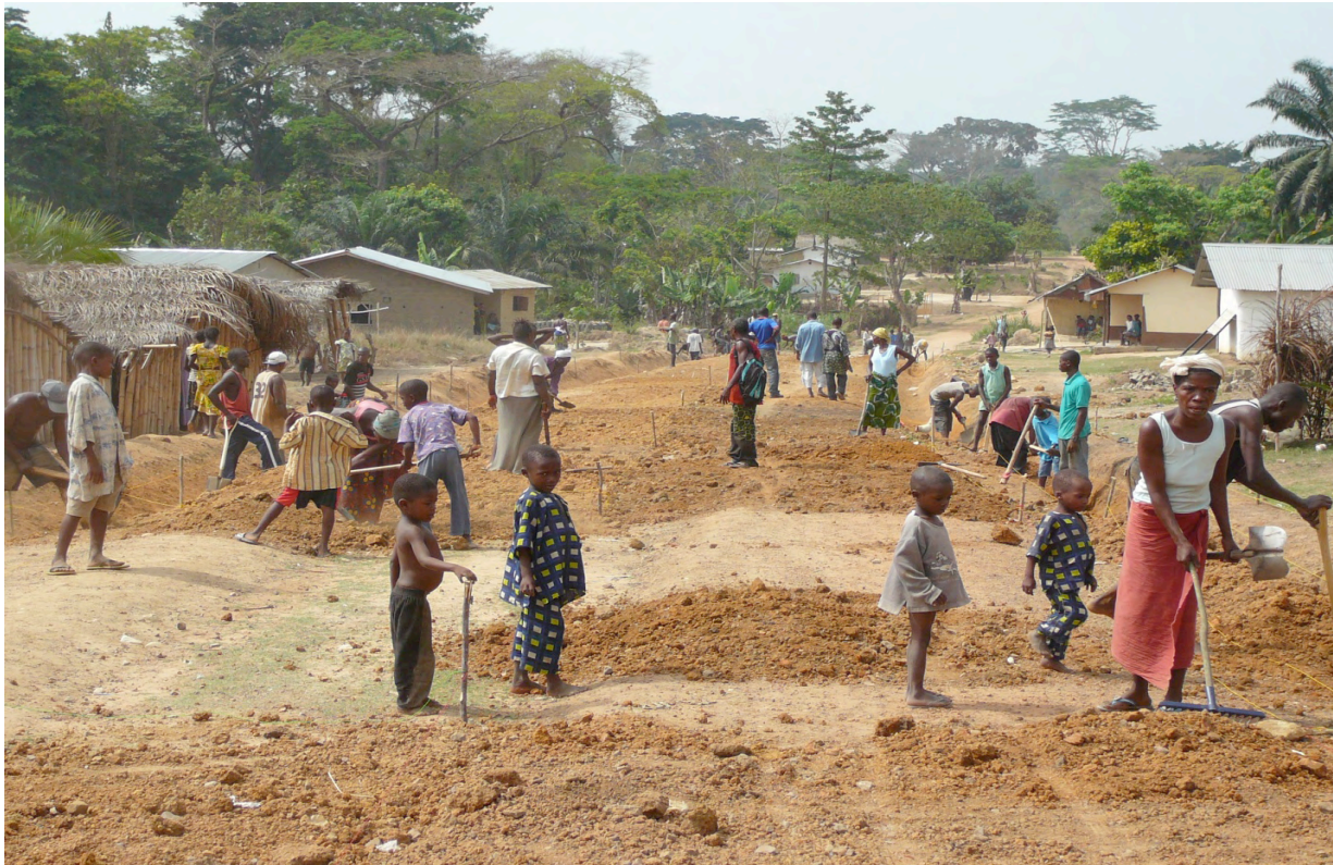
The men dig and the women spread the dirt for the grading that comes later in Phases III and IV.
