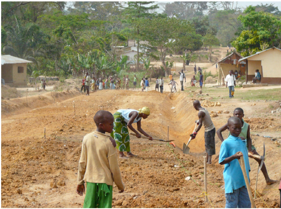
The youth (teens) help and earn also. Compensation finally negotiated was: men would do the heavy digging/trenching at a rate of L15, 000 ($4.00) per 10 meters; and women and youth would do the surface work at a rate of L10, 000 ($2.65) per 10 meters.
