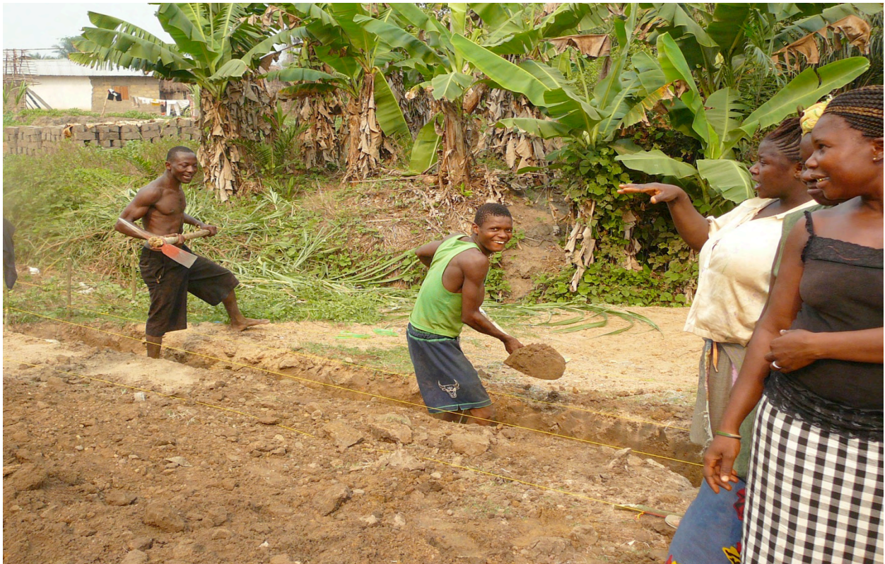
Ditching the road in the Woroma area.
