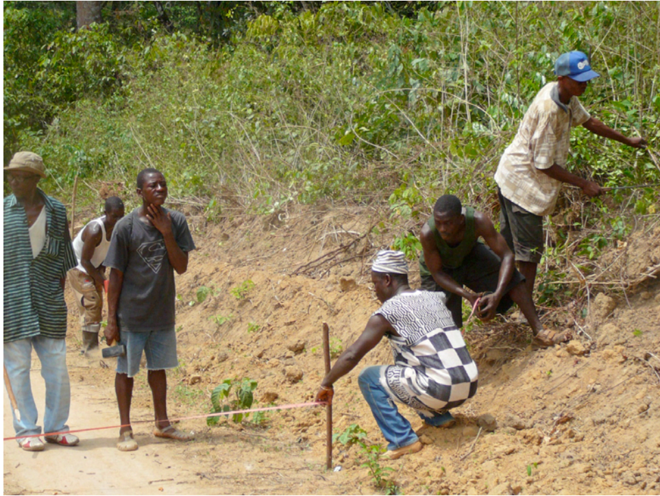
Penguia Paramount Chief Jibilla shows the young workers how to mark the road for ditching.
