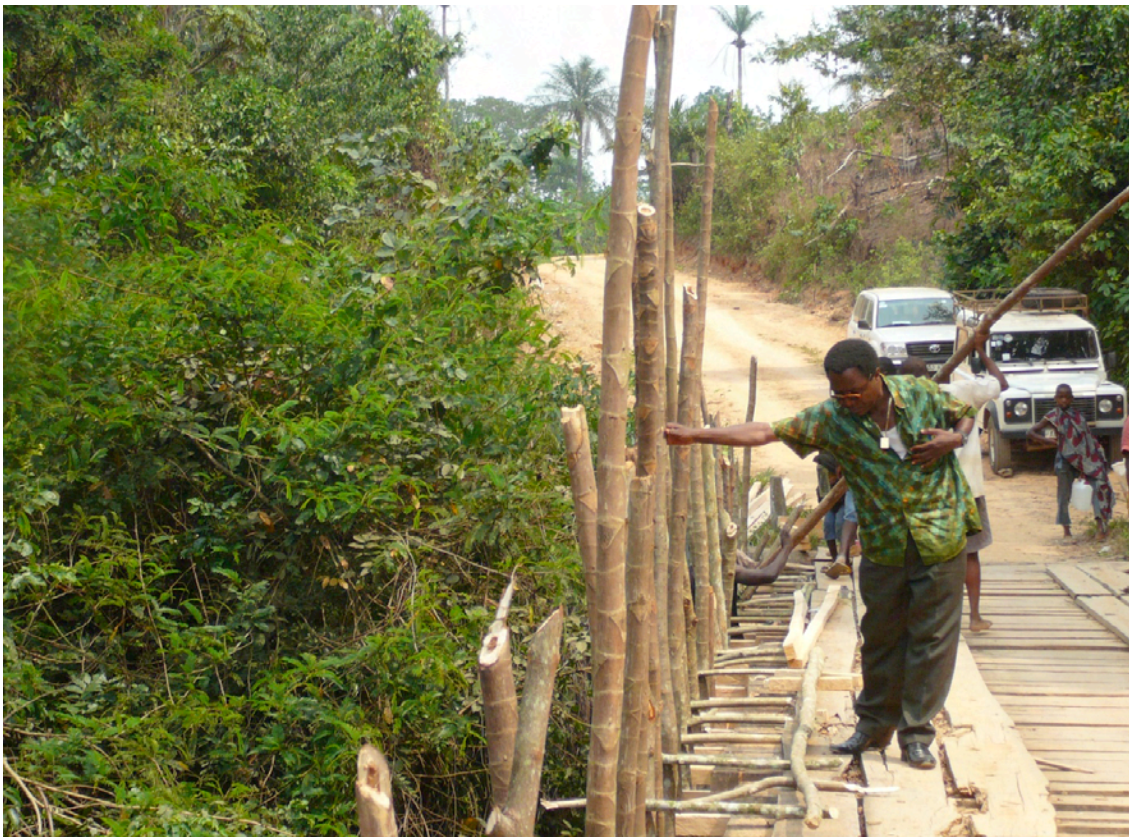
The SLRA Maintenance Director inspects the scaffold installation.
